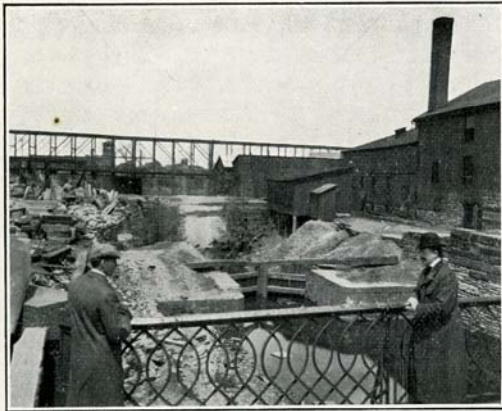
The Abandoned Canal Should be Redeemed and Transformed into a Place for Public Recreation.
